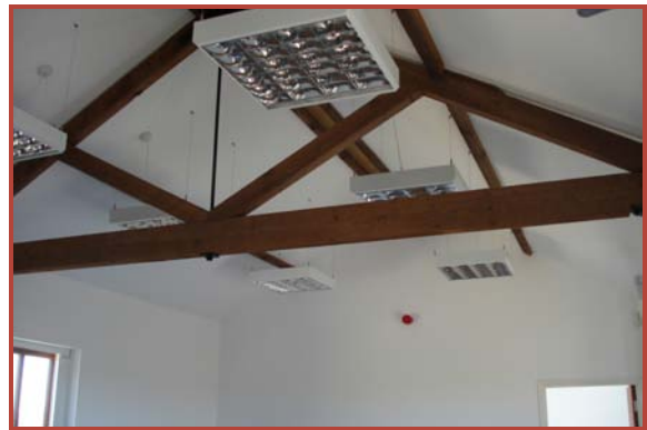
West office exposed beams
