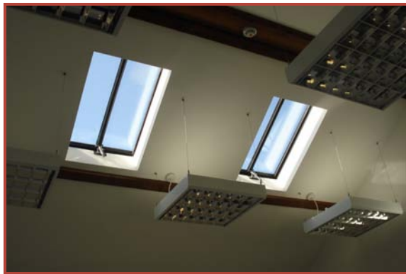
West meeting room skylights
